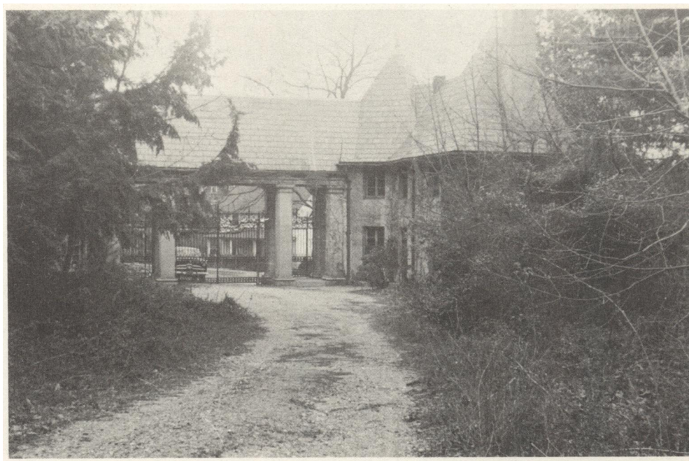
The Gatehouse as seen from within the property when first discovered by the authors.
