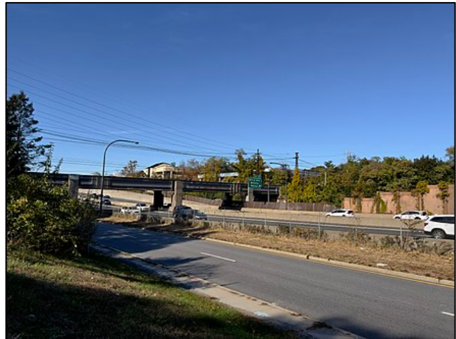
Above: The Long Island Expressway, looking northwest from Parkside Drive and eastbound Powerhouse Road in 2021, showing the Long Island Rail Road overpass. (Image courtesy of Wikimedia Commons)
