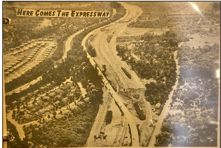
Above: An aerial image from the September 11, 1957 edition of The Roslyn News , showing the Long Island Expressway's construction in Roslyn Heights, looking west. NY 25D is visible crossing the right-of-way. The West Park housing development is visible at bottom-left, and one of the recharge basins can be seen under construction at top-center. (Image courtesy of The Bryant Library Local History Collection, Roslyn, L.I., N.Y. )
