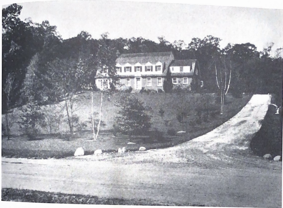
A GRAVEL DRIVEWAY CLIMBS THE SLOPE TO THE STURDY STRENGTH OF THE DUTCH COLONIAL
