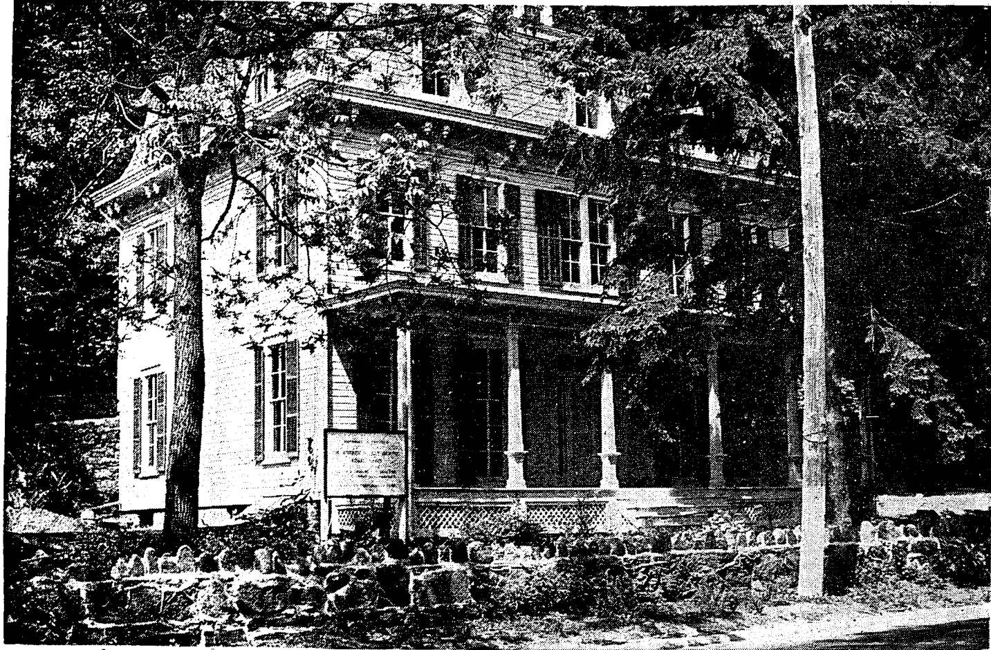
The once-dilapidated Warren Wilkey house, built in the French Second Empire style, has been restored and is for sale.
