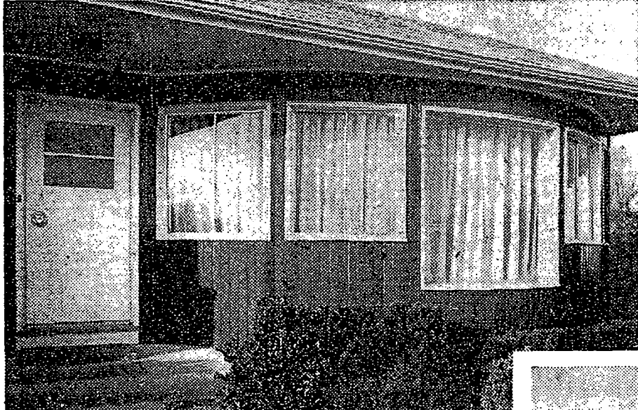
Rounded wall is used by builders, Seidenwurm & Schwartz, as a detail in the new house, whose plan is at right.
